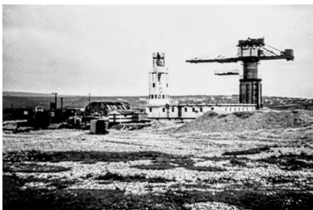
Building took place on the Eastside beach at Newhaven, where the new tower was constructed of concrete in two sections. The base and vertical pillar section were floated into position where the hollow base was flooded and allowed to sink on to a levelled area of the sea bed. The cabin section was then floated out, positioned over the base and allowed to settle on to the column as the tide fell.
